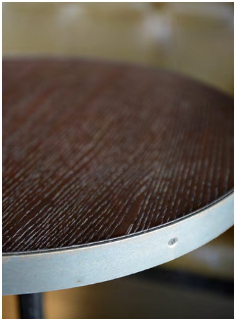
RIFT SAWN WHITE OAK STAINED DARK & CERRUSED W/ STEEL EDGE BANDING AT NOPA - WASHINGTON, DC
